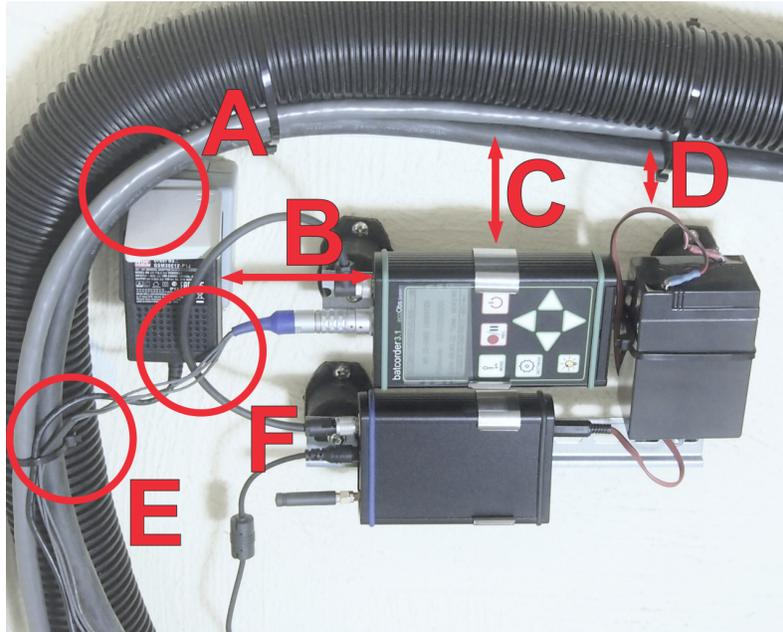
**A:** The 230V socket and thus the power pack are too close to other live lines of the wind turbine.
